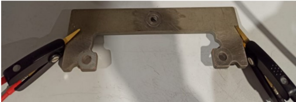
Figure 14: Milometer connected to a copper busbar
